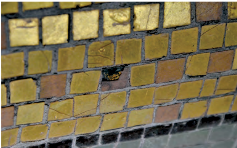
Fig. 1. Altered modern (beginning of the 20 th century) gold glass tesserae, in context (photo B.M. Kürtösi)
