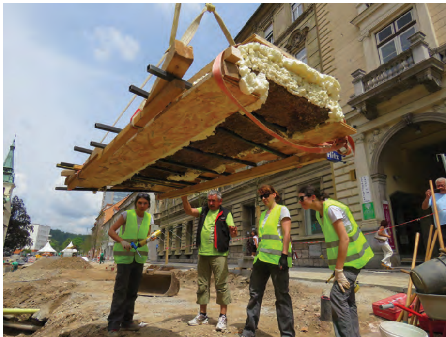
Fig. 1. Lifting the mosaic fragment with all the layers of mortar (photo A. Urbanc)
